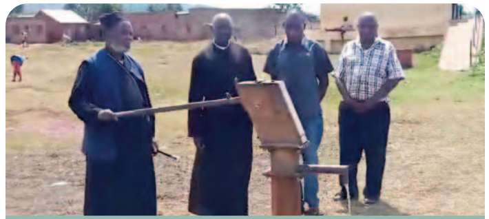
The newly installed water pump and rainwater harvesting system provide clean, safe water for students, staff, and the surrounding community.
